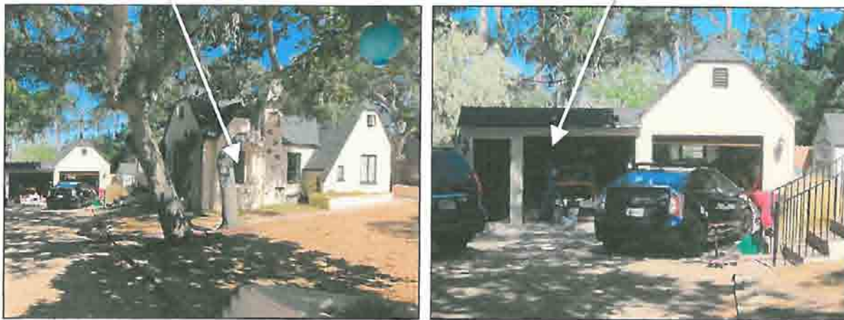
Figures 1 and 2. Two images of the house and garage on the subject property. Left image shows the front elevation of the house with steeply-pitched and jerkin-head roofs, a front-facing chimney, multiple-pane windows and stucco exterior wall cladding. The original entrance was to the left of the chimney on the front elevation (arrow). Right image shows the large addition to the original garage (arrow).
