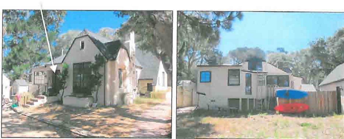
Figures 3 and 4. Left image shows the left side elevation. The original entrance on the front elevation was enclosed and the entrance moved to the side elevation (arrow). The projecting front bay to the left of the chimney was installed when the entrance was moved. Right image shows the large rear addition to the house.
